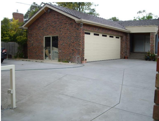
The fully concreted front “garden” is now common-place in Boroondara
